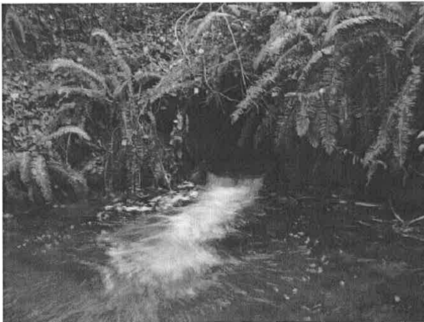
Figure 6.1 Upstream end of reach on proponent's property (culvert under Denewood Pl.)
